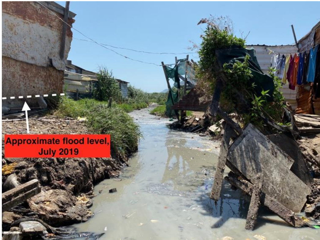
Figure 4. Informal Dwellings and Refuse/Sewage Deposits in Drainage Channels in Wetlands Area (flood-water level denoted by resident) (Author Haley)
